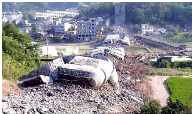
Fig. 10. Progressive collapse of a stone arch bridge in China (image courtesy of Yafang Zhu)
