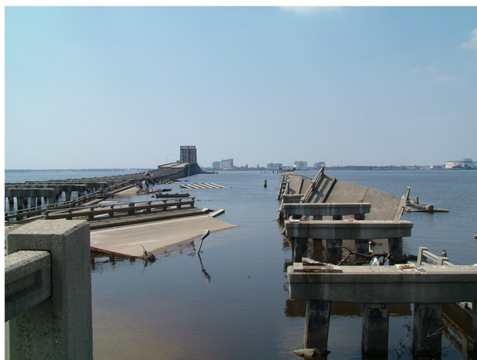
Fig. 5. Bridge decks knocked off pile caps during hurricane (image courtesy of Wikimedia Commons/Joe Furr, WIKIPEDIA 2005)
