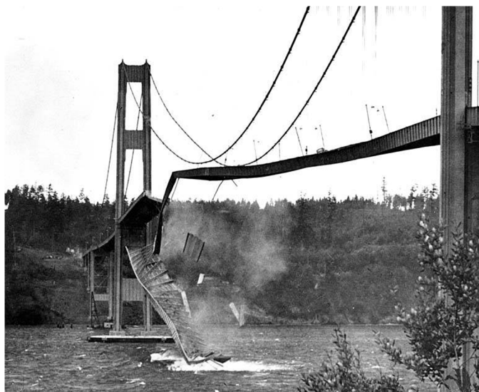
Fig. 1. Collapse of the original Tacoma Narrows Bridge in 1940 (reprinted from WIKIPEDIA 1940 )
