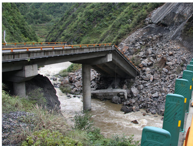
Fig. 4. Collapse of a bridge due to landslide (image courtesy of Xi Zhang)
