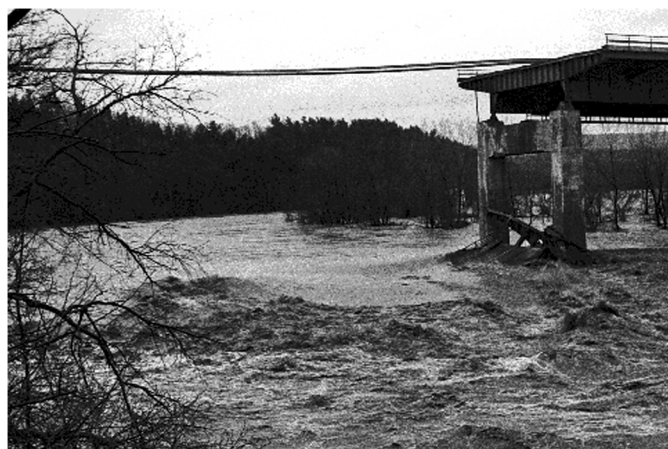
Fig. 3. Collapse of the Schoharie Creek Bridge due to flood in 1987 (reprinted from USGS 2012 )
