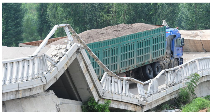
Fig. 6. Bridge collapse due to an overloaded truck (image courtesy of Yuqiang Liu)
